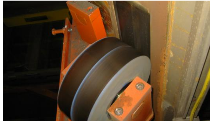
Floor-to-floor elevator guide wheel of NYTEC-HS
